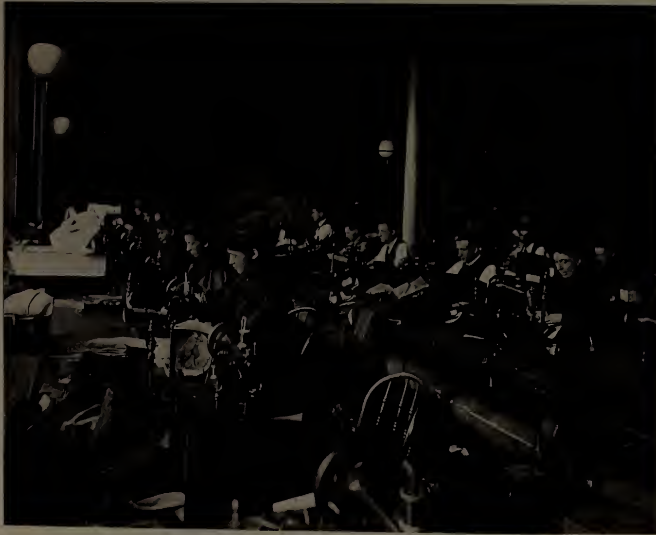
MACULLAR PARKER COMPANY. One of the Workshops, 400 Washington Street.
